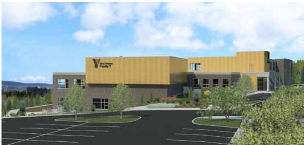
View From The Northeast
